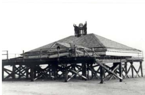
Men atop a the roof of the collapsed Boardwalk Pavilion in Margate after the 1962 Ash Wednesday Nor'easter.
